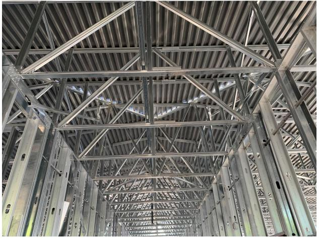
The photo above was taken in the eighth grade hallway and if you look closely you can see the area where the slopes transition. The camera is facing north. The water on the sheets directly above the camera will flow south. Water on the sheets north of the light line will flow east and west. That conversation will be much easier to follow after the rest of the roof sheets are installed. After the roof is completed, there should be no water making contact with the sheets in the picture.
