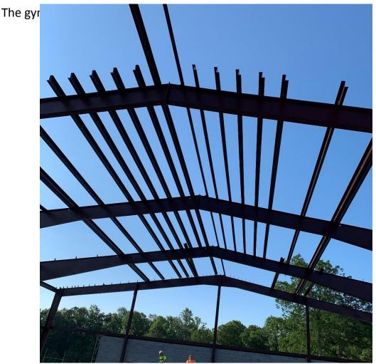
Most of the purlins have now been installed. They seem narrowly spaced near the center of the roof but somebody felt they were necessary.
